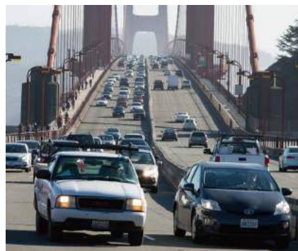
Bridge Security Checkpoint
